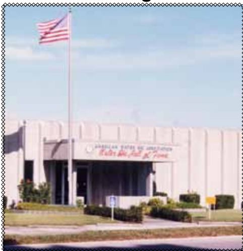
Preview Center, Overlook Drive location
